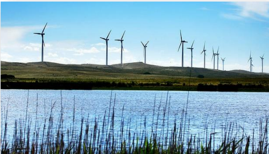
Figure 2- Wind farm western Victoria - Jessica Shapiro
